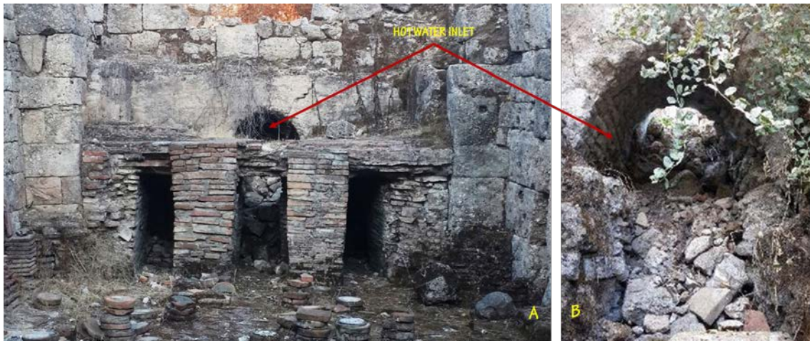
Fig. 18. a. Caldarium Hypocaust System , b. Hot Water Pool Water Inlet
