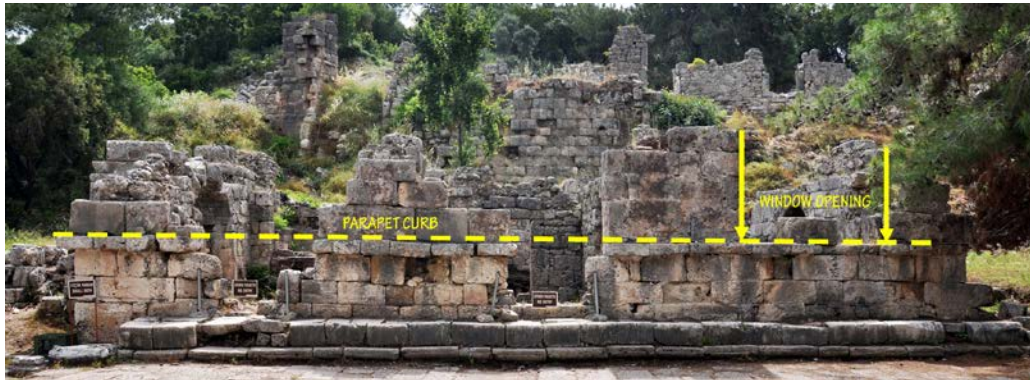
Fig. 11. Border and Frigidarium Window Opening Along the Entire Facade
