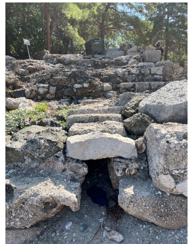
Fig. 18. Discharge Area of Drainage to Central Harbor
