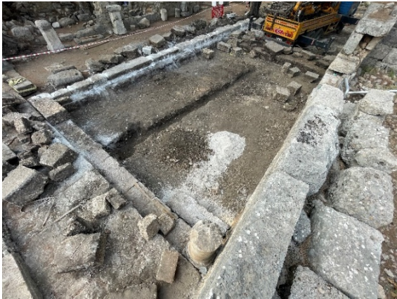
Fig. 10. Main Drainage System Excavation Aerial View
