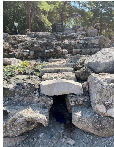
Fig. 18. Discharge Area of Drainage to Central Harbor
