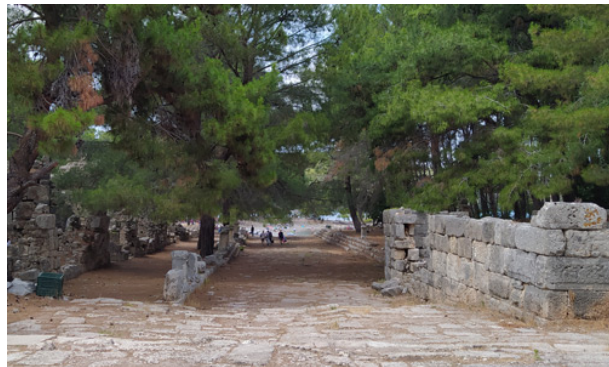
Fig. 8. Main Street View from the South before Conservation Work
