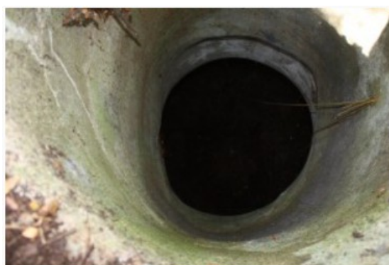
Fig.2. Cistern 1.S.2. (Kürkçü 2015, 76)
