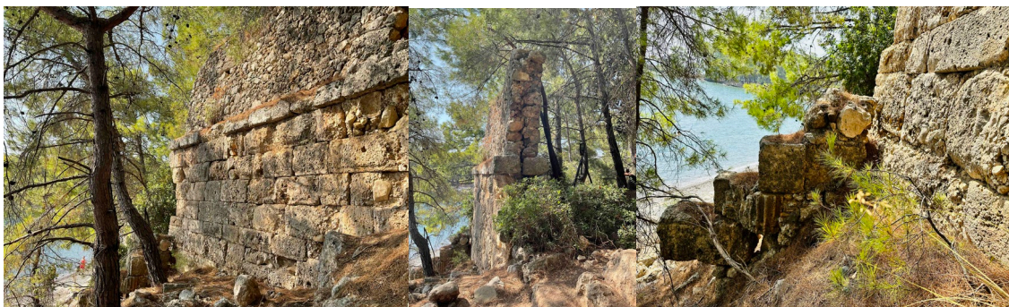
Fig. 9. Water Route Found in the Northern Necropolis Area (Cesur 2024, 71)
