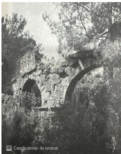
Fig. 5. Phaselis Aqueduct, G. Bean 1968
