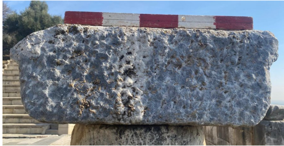
Fig. 4. Column Capital from the Theatre ( Proskenion , First Story)
